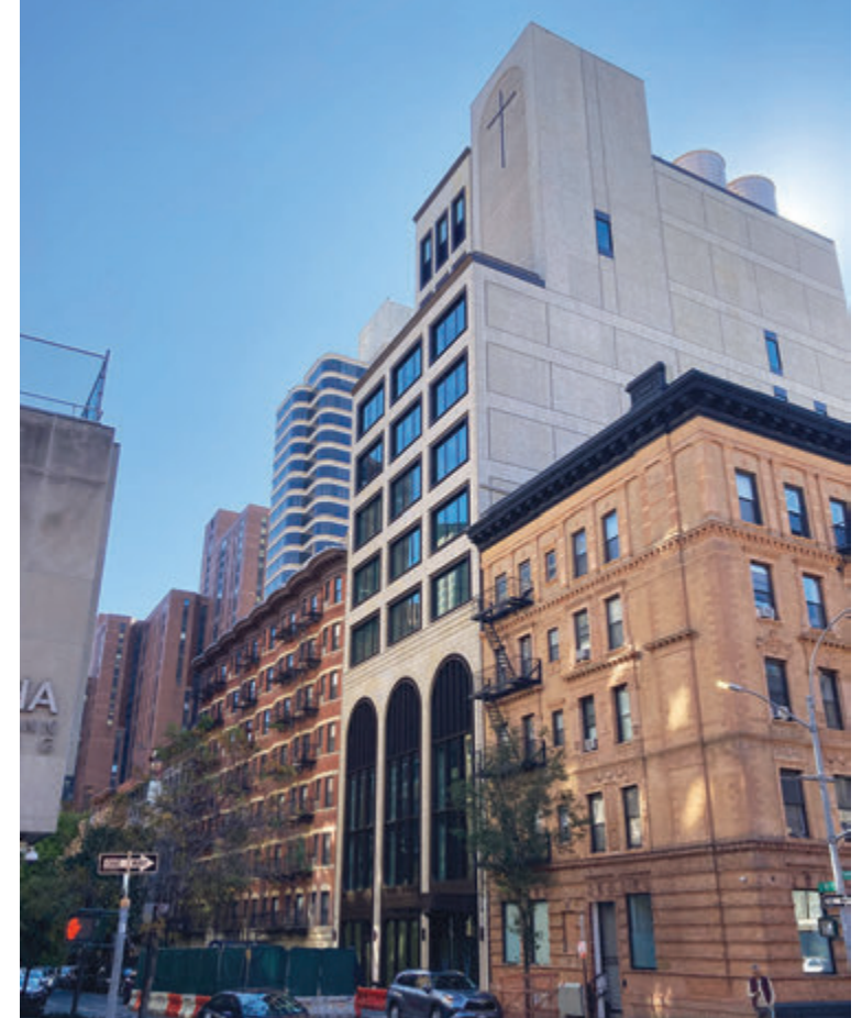
CONSTRUCTION OF MID-BLOCK CHURCH NEARS COMPLETION In 2022, we learned that the East 91st Street Christian Church had acquired a 50-foot-wide, six-story apartment building, which was demolished. In its place now is an 11-story ministry center including worship and assembly halls and 17 classrooms. While the height and design stand out from its surroundings, it was built as-of-right. Its tall cross is inlaid at the top floors and blends in with the upper facade.
